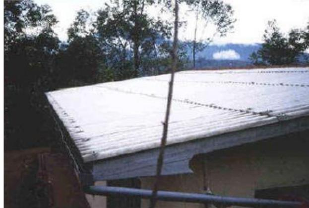
Figure 2: Typical Corrugated Iron Roof, Photo: Practical Action
