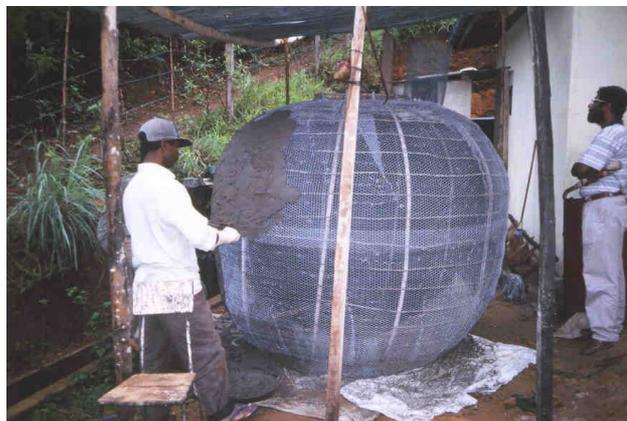
Figure 12: Construction of Pumpkin water tank in Sri Lanka
