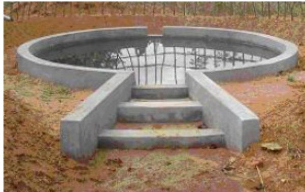
Figure 14: Runoff rainwater harvest tank
