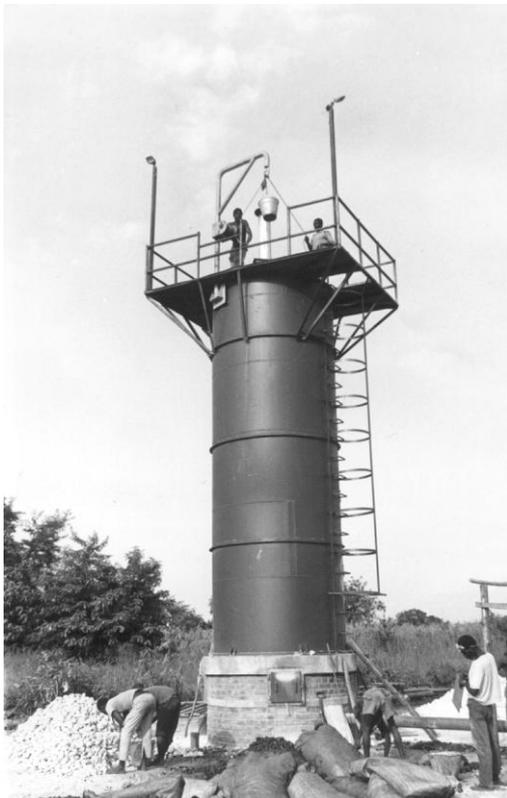
Figure 1: The improved kiln design.
